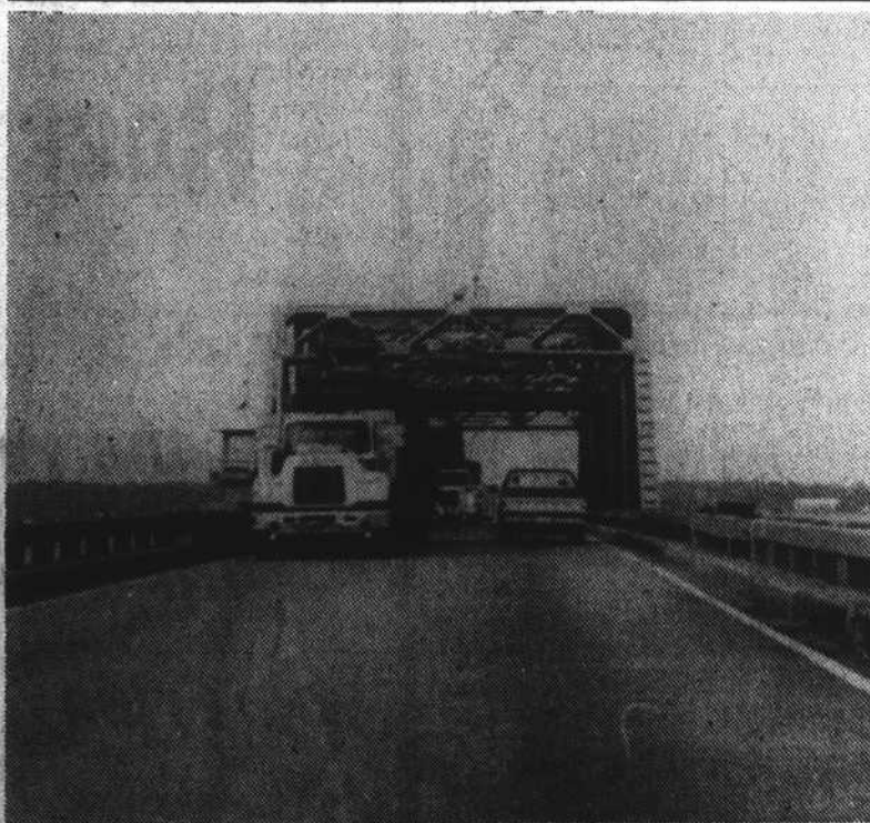
CLOSE CALL —The draw across Chowan River Bridge has been beset with problems when over-height trucks and equipment try to squeeze through and hit the span. The bridge had another close call Monday around 7:30 p.m. when the truck in the front cleared safely, but the one in the rear was almost too tall. The truck slowed to a crawl to prevent bouncing and squeaked through the opening.
