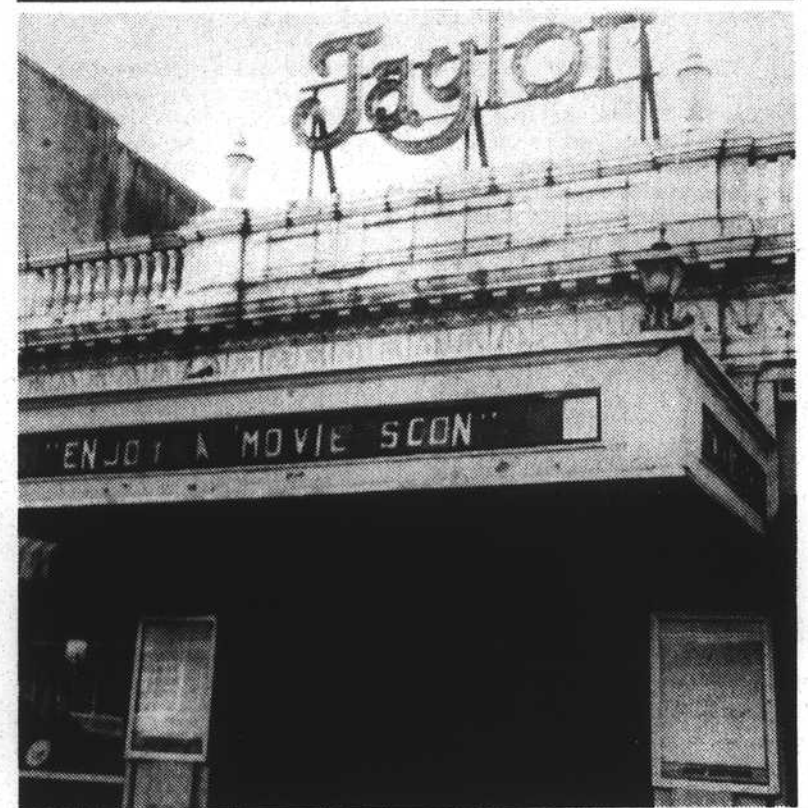
"CLOSED UNTIL FURTHER NOTICE"—That sign replaces movie billings that have flanked the entrance of the Taylor Theater on Broad Street since 1925. Wilson Amusements, until Sunday, operator of the theater, sees no future for the business. Owners, Mr. and Mrs. W.J.P. Earnhardt, are not so pessimistic and expect to see it reopened.
