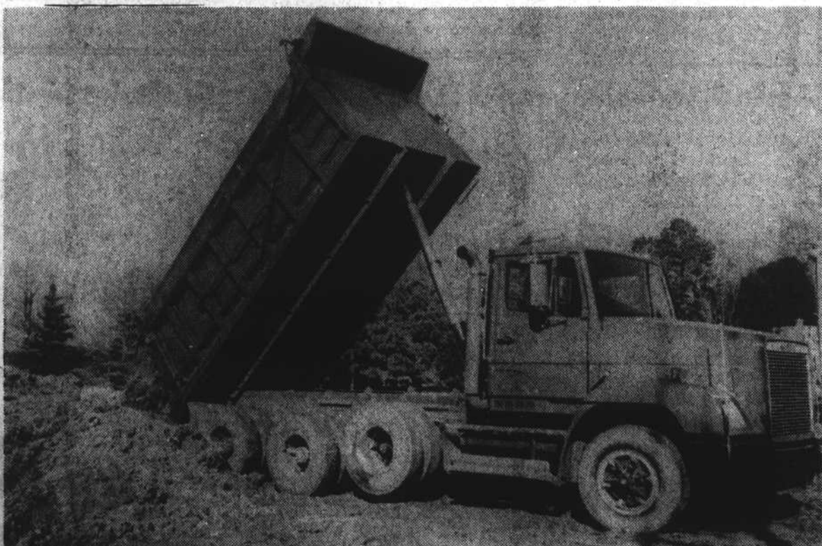
DELIVERED - A large dump truck delivers the last of 30 loads of good topsoil to the new park site behind the Edenton Police Station. A contracting company donated about 100 truckloads to the town at an estimated value of $8,000. The remaining loads went to a fill area at the cemetery. The contractor, McDevitt and Street of Charlotte, excavated the dirt during construction of the new Food Lion store at the Edenton Village Shopping Center. The company said that it was not cost effective to try to sell the soil.
