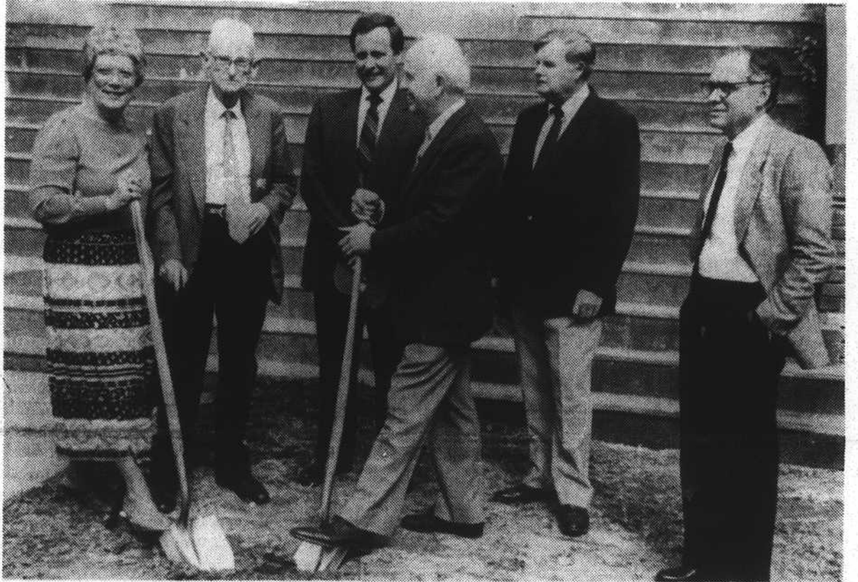
GROUND BROKEN -Ground was broken last week for the conversion of Swain School into apartments and renovation of the auditorium into a center for the arts. Doing the honors were (l. to r.) Clara Boswell, county commissioner, Ernest A Swain, retired educator and the school's namesake, Edenton Mayor John Dowd, Alton Elmore, county commissioner, Roy Mannis, president of W.H. Weaver Construction Co., and Dwayne Anderson, developer.
