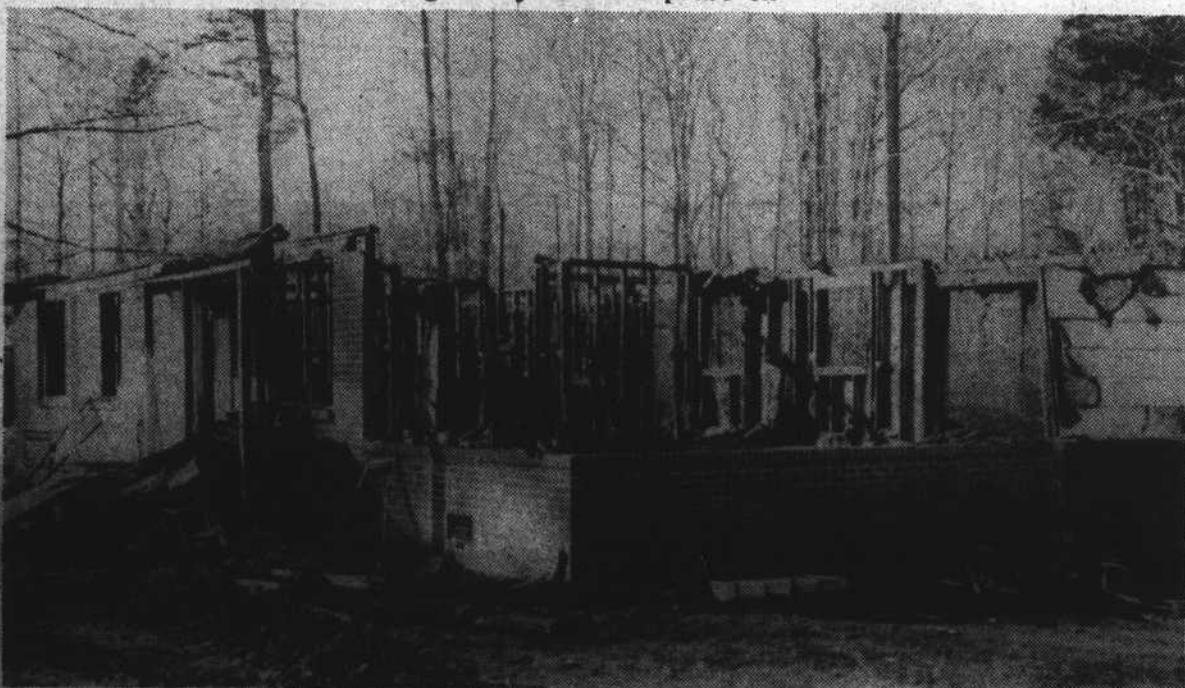
DESTROYED--The extent of the damage is apparent to the golf pro's residence at Chowan Golf and Country Club in a fire that occurred early on Nov. 30. The near side where the fire is believed to have been set shows near total destruction.
