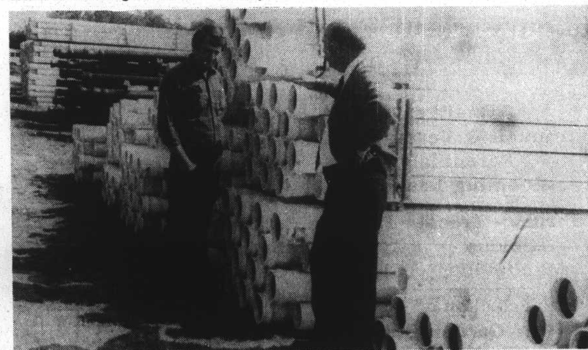
MILES OF SEWER PIPE -- Associate Superintendent of Schools James Kinion (right) and Norman Range, construction superintendent, discuss the many construction projects underway for the schools. They are shown with sewer pipe stacked at Chowan Middle School earlier this month. The pipeline project, started in late April, will connect Chowan and White Oak Schools to the Edenton sewer system. Chowan will be connected by about 12 miles of 6 inch pipe while a 4 inch line will join with it from White Oak. The line installation is rapidly progressing down N.C. 32 North in the $583,000 project.
