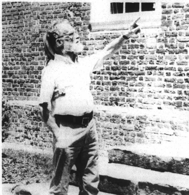
Phase I work was completed on the 1767 Chowan Courthouse
