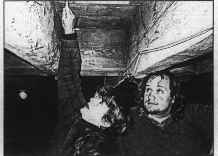
Linda McNaughton and Tom Beaman (above) point out the tool marks in the hand hewn beams that make up the old Chowan County Courthouse foundation. (Staff photo by Helen Kerr Outland)
