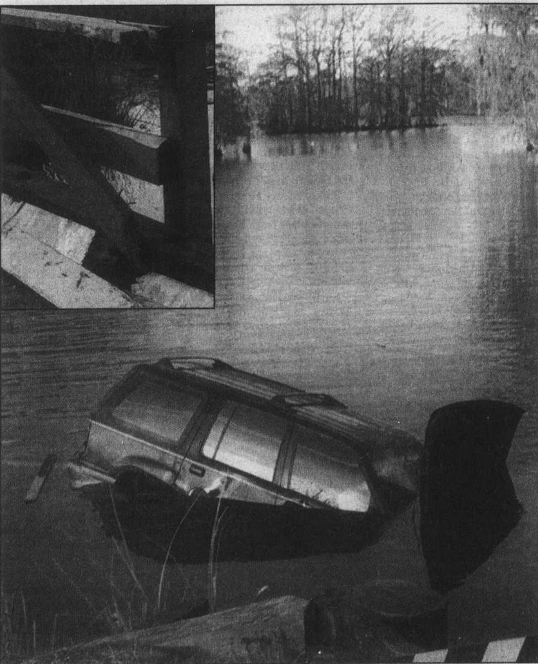
The female driver of this vehicle sustained only minor injuries Thursday morning when her car left the road and crashed thru the railing of this bridge on Rocky Hock Creek Road. The teenager was charged with failure to maintain lane control. The eight foot span of railing was replaced by day's end. (Outland Photo)
