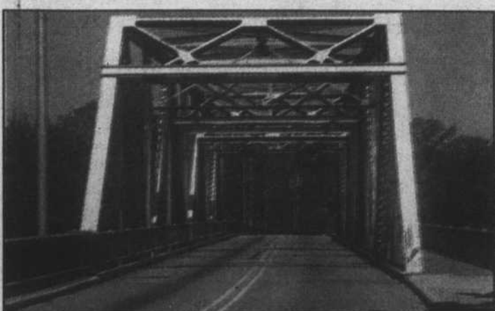
The Perquimans River Bridge is slated to obtain lights as part of the streetlight enhancement project.
