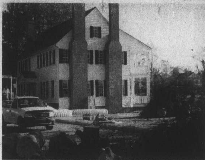
The Barker House suffered the most serious damage of any historic site in Edenton. (Staff photo by Bud Weagly)
