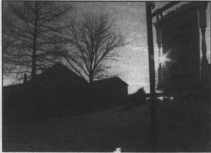
Town Manager Anne-Marie Knighton says she'll keep pressing FEMA to reimburse Edenton for funds needed to repair hurricane damage to the Northeast Partnership building rather than support a recommendation from the NC Local Government Commission staff to raise local taxes to pay for the work. The Partnership building is owned by the Town of Edenton. (Staff photo by Sean Jackson)
