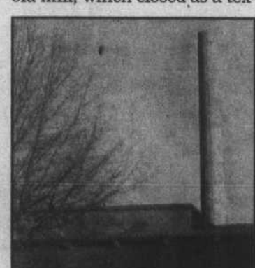
Designers for the Edenton Cotton Mill plan on removing an undetermined portion of the mill's chimney.
