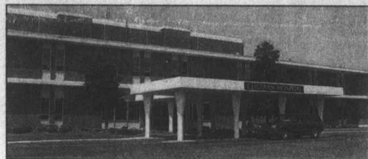
Chowan Hospital is now a critical access care facility.
