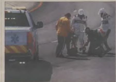
Workers patch an area of track pavement at New Hampshire Motor Speedway during a break in the action Sunday.
