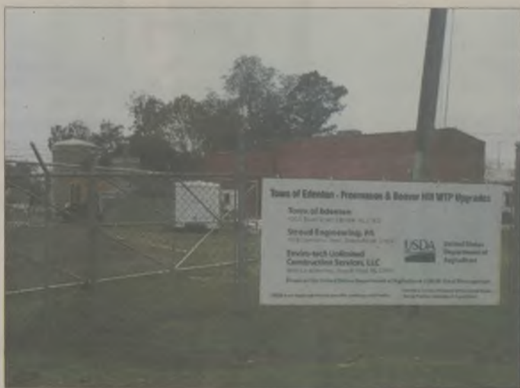
Upgrades to Edenton's Beaver Hill Water Treatment plant were recently completed.
