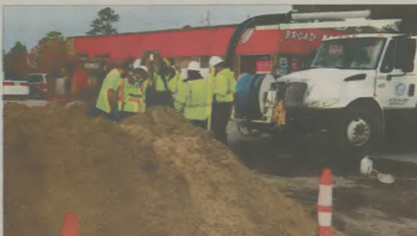
Edenton Public Works staff works to repair a sewer line leak.
