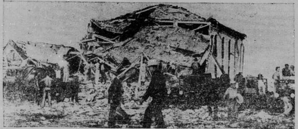
Amid crumbling masonry and steel, rescue workers and frantic parents hunt for bodies of children killed and mangled by explosion.
