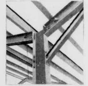
Detail of roof connections at column.
