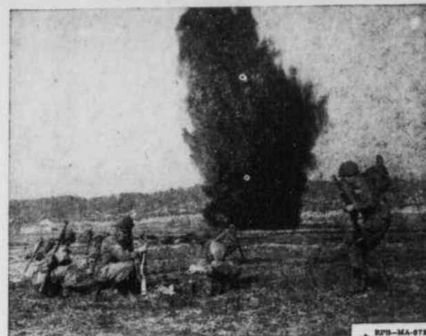
This 11th Airborne Division demolition crew in Japan has just detonated a charge of explosives in blowing up a bridge during tactical training courses. These men are receiving the finest training available, and will become efficient, well-trained soldier-specialists. Men on occupation duty, as well as elsewhere, have excellent opportunities for careers with a future in the U. S. Army.
