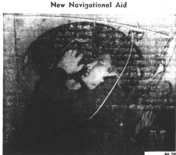
It's a bubble octant. This United States Air Force student at Ellington Air Force Base, Texas, is taking a peek through the new device as part of his navigational training in the AF's new Consolidated T-29 Navigation Trainer.
