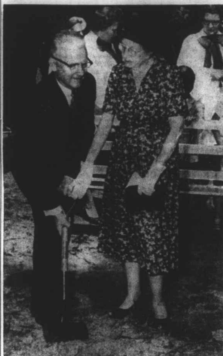
GROUND BREAKING CEREMONIES were held at the Andrews Presbyterian Church Sunday. Beginning operations for the new church educational building are starting this week. L. B. Nichols, ruling elder, and Mrs. C. A. Brown, oldest member of the church present, turned the first shovel of earth for the construction. (Photo by Smiley Studio)
