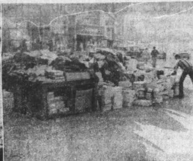
FIRE DAMAGES ETHEL'S SHOP
