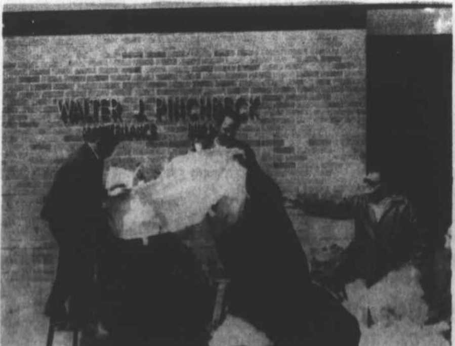
THE WALTER J. PINCHBECK MAINTENANCE BUILDING ON THE PSU CAMPUS.
