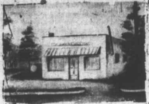
POST OFFICE BOX 1075
