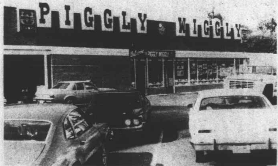
Pembroke Piggly Wiggly. The Drose family speaks highly of Adolph Dial, the landlord and builder of the 11,500 square foot store, modern in every respect. Said John Drose, Jr., "Mr. Dial has been as
