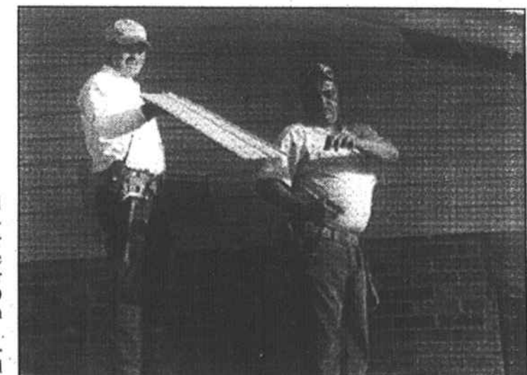
James "Rooster" Smith (left) and Milton Cummings install soffit at a unit in Chavis Park.
