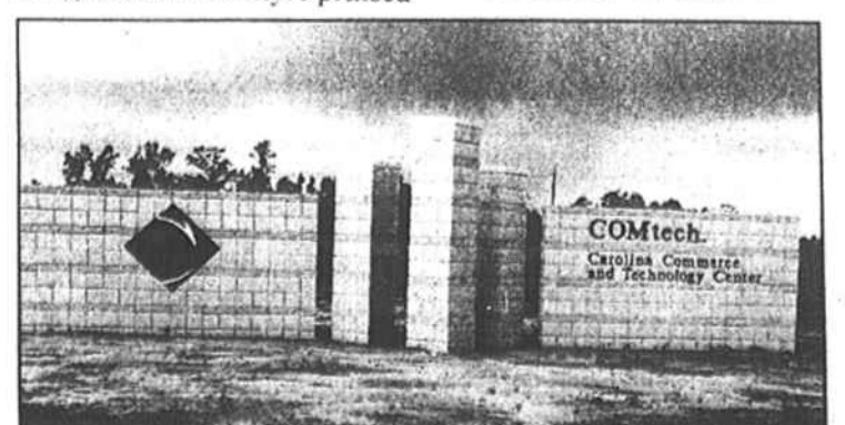
The entrance to COMtech or, more correctly, "Carolina Commerce and Technology Center"
