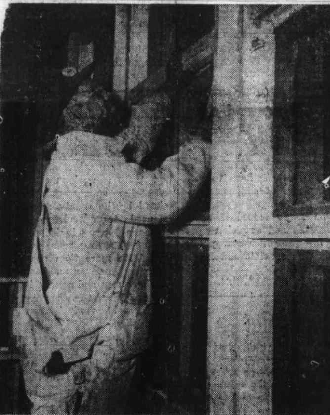
One of the 600 skilled workers employed in the construction of Wake and Midway Halls, new dormitories for 1,000 Negro women war workers in Washington, D.C. The million-dollar job was recently completed by Samuel Plato, Negro contractor.
