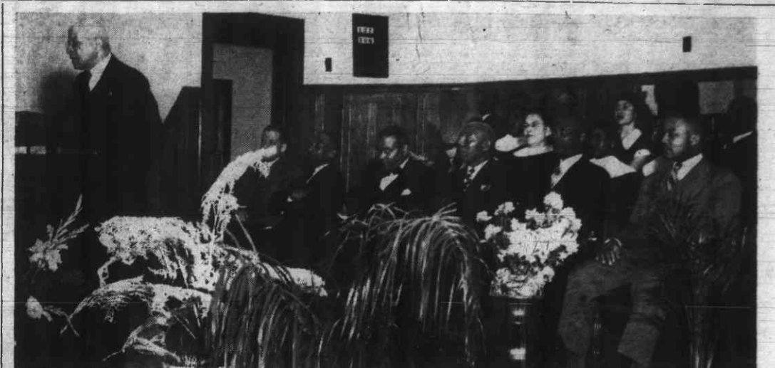
The new Saint John Baptist Church, located on Third Street here in Durham, was formally opened last Sunday with dedicatory services at two o'clock. The new church building was erected at an approximate cost of $60,000. Work on it started in February, 1949, and was completed early last month. In the above scene, Dr. C. C. Spaulding, president of the North Carolina Mutual Life Insurance Company, is shown (standing) delivering one of the featured addresses at the afternoon service.
