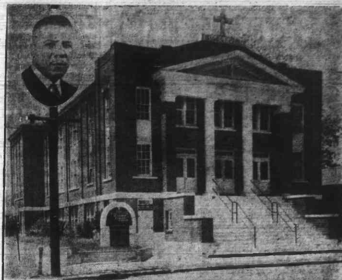
The First C. M. E. Church of Montgomery, Alabama recently completed a $3,500 renovation front of the church to the base. A complete concrete floor was put in the entire basement. Dr. R. O. Burtley is the progressive pastor. The Right Reverend B. W. Doyle, presiding Bishop.
