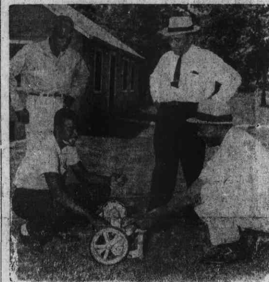
4-H'ER MAKES POWER MOWER —MacArthur West, an 18-year-old 4-H Club youth of Clarksville, Tenn., is getting his homemade power mower ready to be put on display in his community during National 4-H Week, March 4-11. The youth converted his old hand mower into a power mower by a tach-
