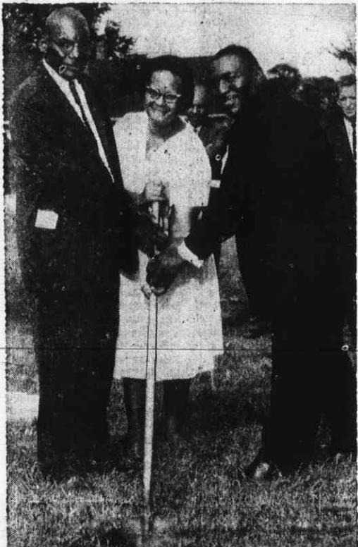
GROUND BREAKING CEREMONY Shown left to right as they break the ground at the site on which the new Mt. Calvary Holiness Church is to be erected are: Willie Robinson, superintendent of Sunday School, and a member of the building committee; Mrs. Isabel Dunn, a donor, and Bishop F. Yelverton, pastor. The ceremony was held Saturday, September 19.
