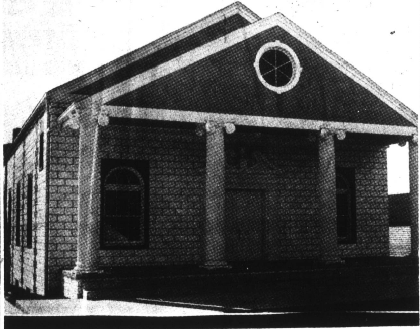
THIS IS THE EBENEZER BAPTIST CHURCH building on Gillette St. in East Durham which is to be torn down to make way for the new east-west expressway.—The last services are being held here Sunday, July 28, morning and evening. A new church is under construction. (See picture on page 4A)
