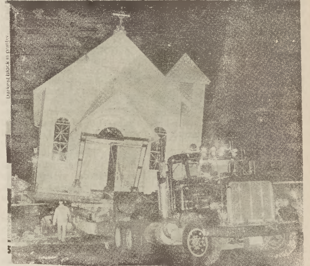
KALAPANA, HAWAII — Volunteers work from throughout the night to load the Star of the Sea Painted Church on to a truck in hopes of moving the historic church before lava from the Kilauea volcano moves in. Over 130 structures have been lost to the lava so far. (UPI Photo)
