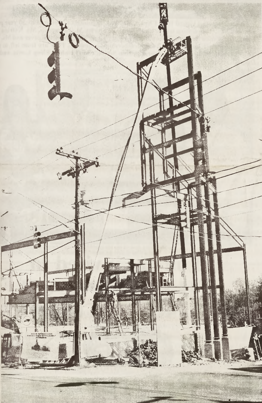
First Calvary Baptist Church at the corner of Kent and Morehead Avenues taking shape. The new edifice will replace the old building. The church worships at 2000 Lakewood Avenue in Lakewood Shopping Center. (Photo By Lawson)
