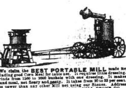
We claim the BEST PORTABLE MILL made for grinding good Corn Meal for table use. It requires little dressing. Grinds from 1860 to 2000 bushels with one dressing. It makes round meal, not flowry and pasty. It takes from 20 to 23 per cent. less power than any other Mill not using our Stones. Address BBANOH OFFICE NORTH CAROLINA MILL STONE CO., Charletts, R. C. Cha nov23-d
