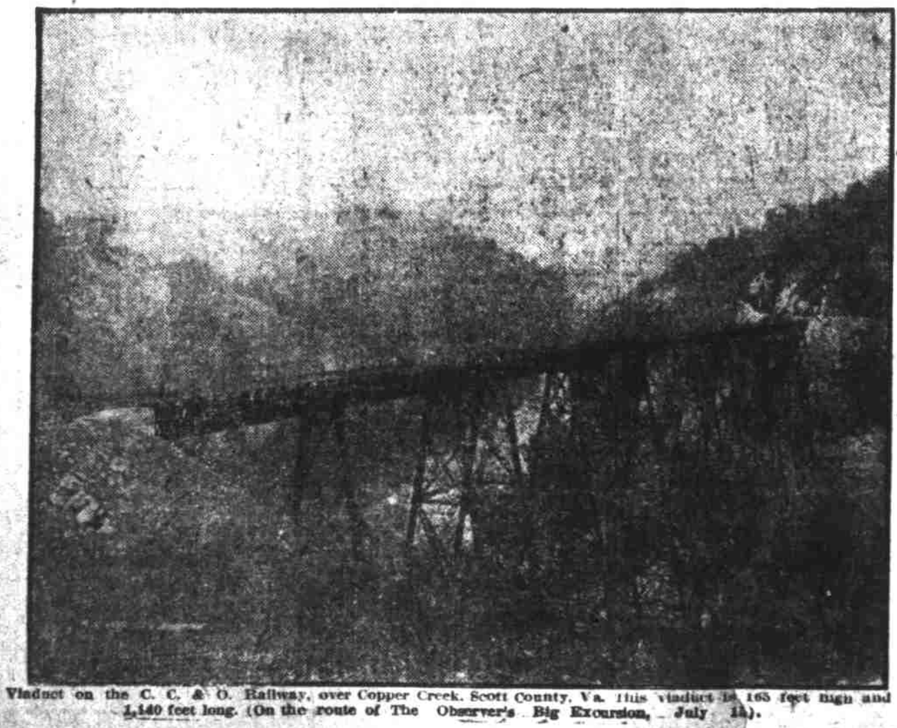
Viaduct on the C. C. & O. Railway, over Copper Creek, Scott County, Va. This viaduct is 163 feet high and 1,140 feet long. (On the route of The Observer's Big Excursion, July 15.)
