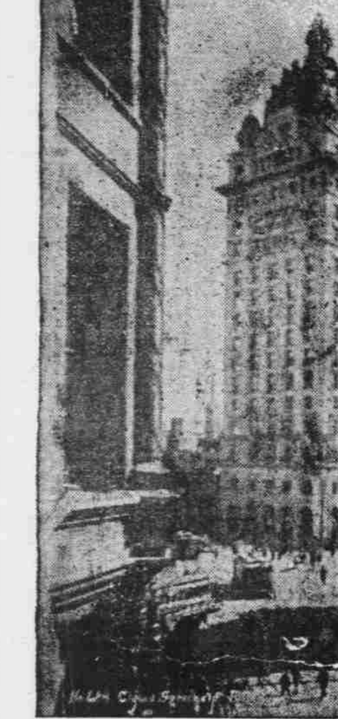
THE CALL BUILDING, ALSO DESTROYED.
