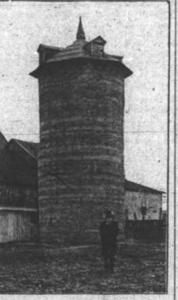
Silo on a Southern Dairy Farm.
