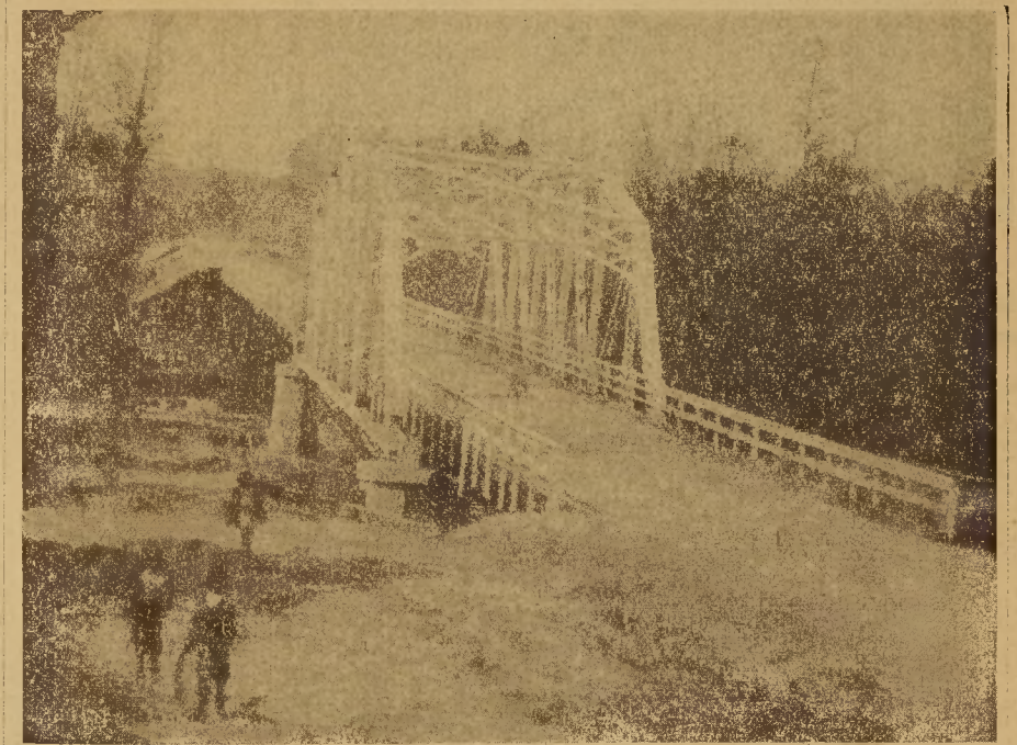
SYMBOL OF A NEW ERA —The modern lines of a steel bridge spanned Meherrin River at Murfreesboro in the late 1920's, replacing an old timber bridge which had served in the days of the horse and buggy. The bridge joined a wooden causeway (background) across low ground on the Maney's Neck shore. Timber from the old wooden bridge was used in houses built in
