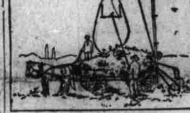
Derrick for Loading.
