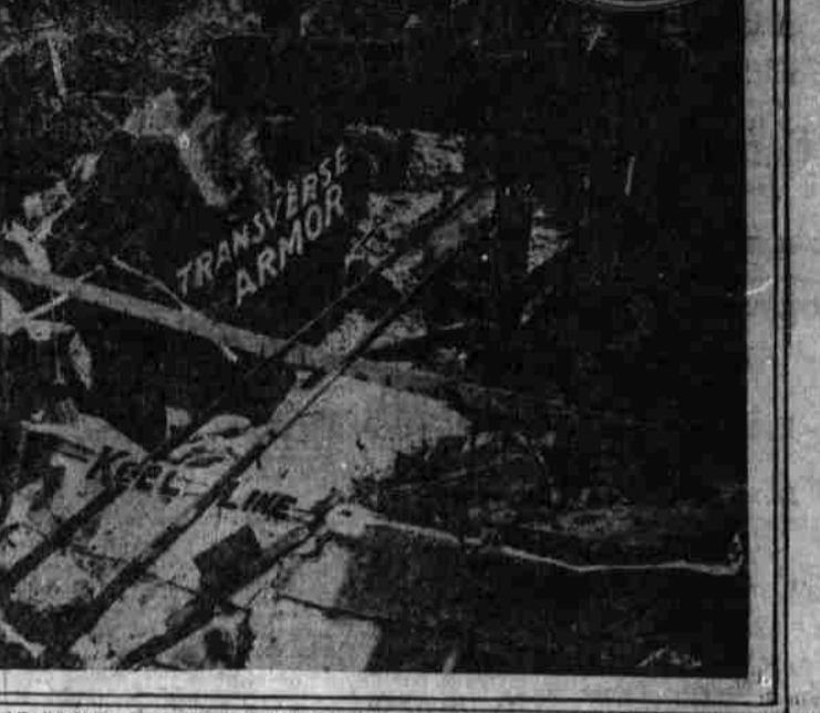
PHOTOGRAPH OF MAINE WRECK, SHOWING FRAME 30 UNDER WHICH BOARD SAYS FIRST EXPLOSION CAME.
