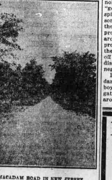
MACADAM ROAD IN NEW JERSEY.
