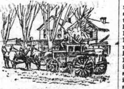
UNDRAINED DIRT ROADWAY. (From Good Roads.)
