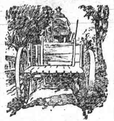
RUTS RUIN THE ROAD.
