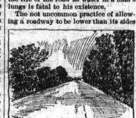
MORE LIKE THIS REEDED. nakes it little better than a mere drain for water settles on the surface, quickly softens it and prepares it to be cut up by every passing vehicle. A raised and crowned roadbed which will shed water readily is essential. A dry base with a slightly arched cover of stone capable of
