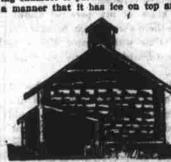
TORROTHE AND COOLING CHAMBER. on three sides. The dimensions are 12 high, with a cooling chamber parti-tioned off 8 feet long by 6 feet wide. The floor of a cooling chamber should be placed about three feet below the surface of the ground so as to take ad-vantage of the coolness of the earth.
