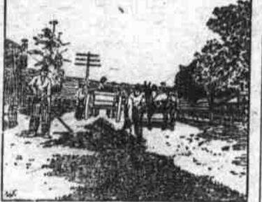
REPAIRING A ROAD.
