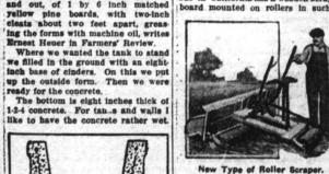
way that it can be raised or lowered as the operator rides he can dig into the ground, or deposit earth as re-quired, simply by manipulating the levers. The trailing rollers not only smooth down the earth, but make the pulling easier for the horses.-Popu
