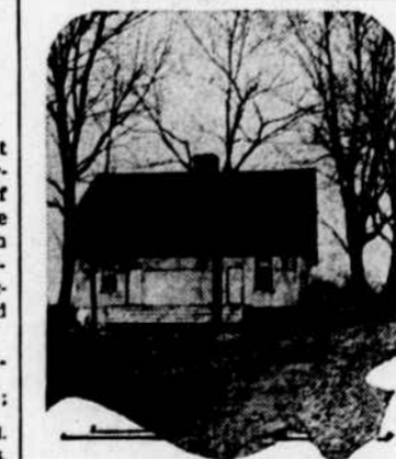
It was in this structure, according to Revolutionary historians, that General Washington made plans and issued orders for the successful conduct of the decisive victory at Trenton.
